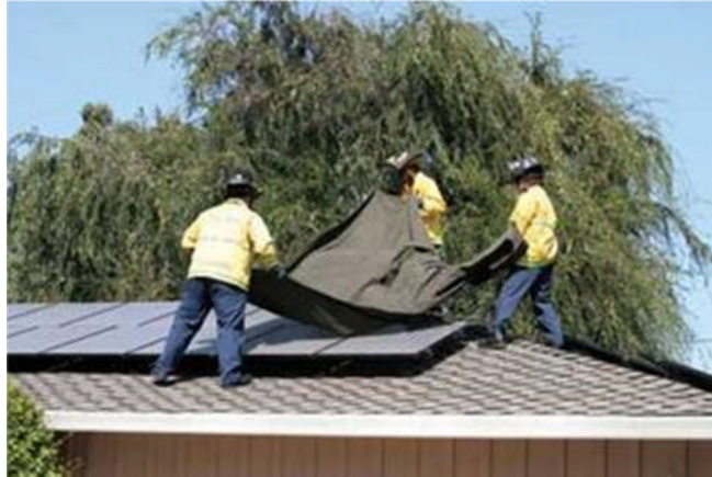
Photo 5. Tarping an array to make it electrically safe.
