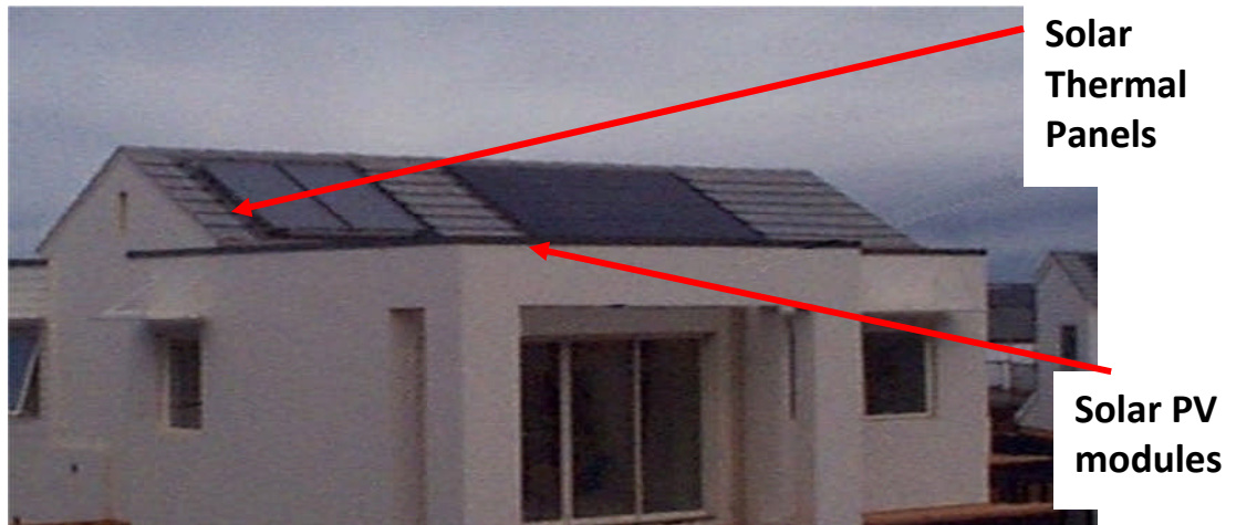
Photo A3. House in Sydney Olympic Village Sydney with both solar thermal and solar PV electric panels
