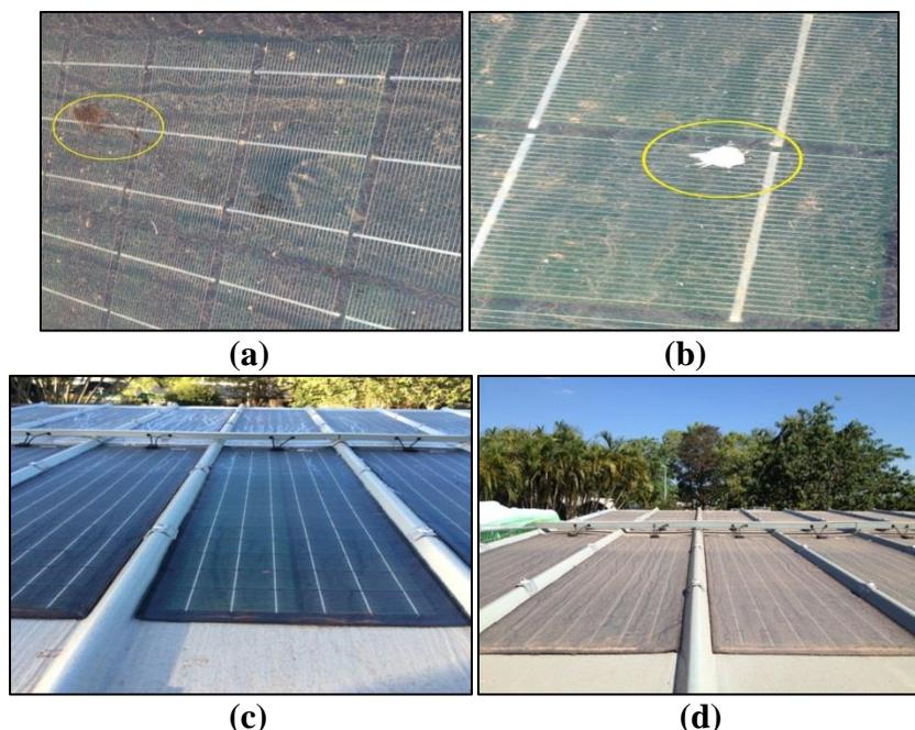
**Figure 7: (a) Surface with bat droppings, (b) Surface with bird droppings, (c) Clean modules after morning dew, (d) Natural dust accumulation**
