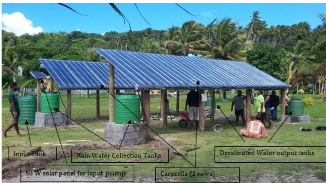
**Fig 4.2: Construction of the Desalination system**
