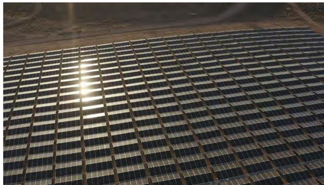
**Figure 1: East-West high ground coverage ratio solar farm**
