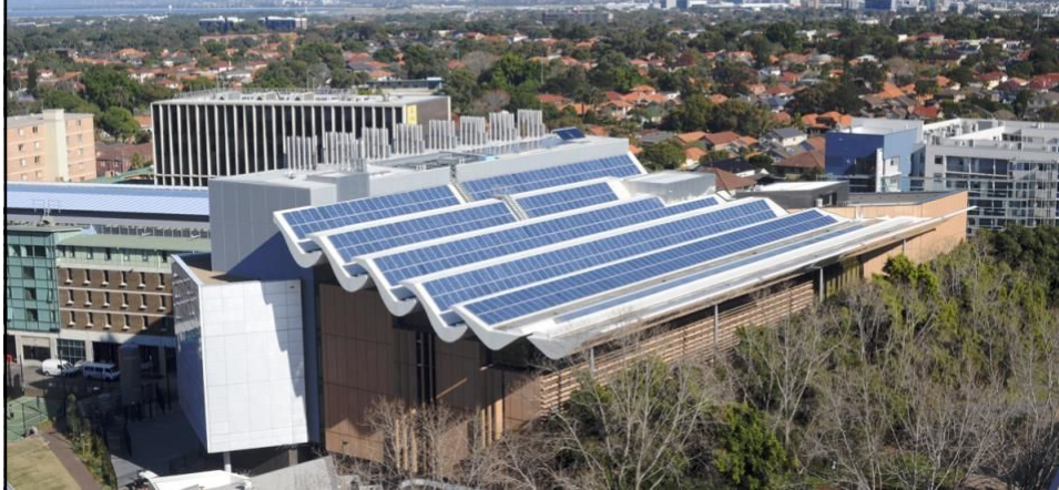
150kWp Tyree Energy Technology Building, UNSW
