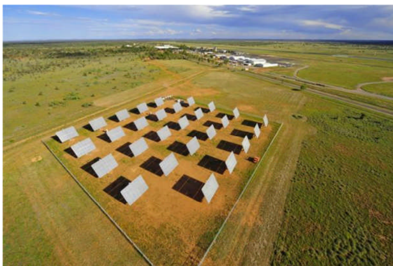
Alice Springs Airport 235kWp PV System (photo courtesy Alice Solar City Project).
