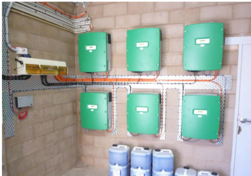
Grid-connected inverters in a commercial rooftop PV system in Alice Springs (photo courtesy Alice Solar City Project).
