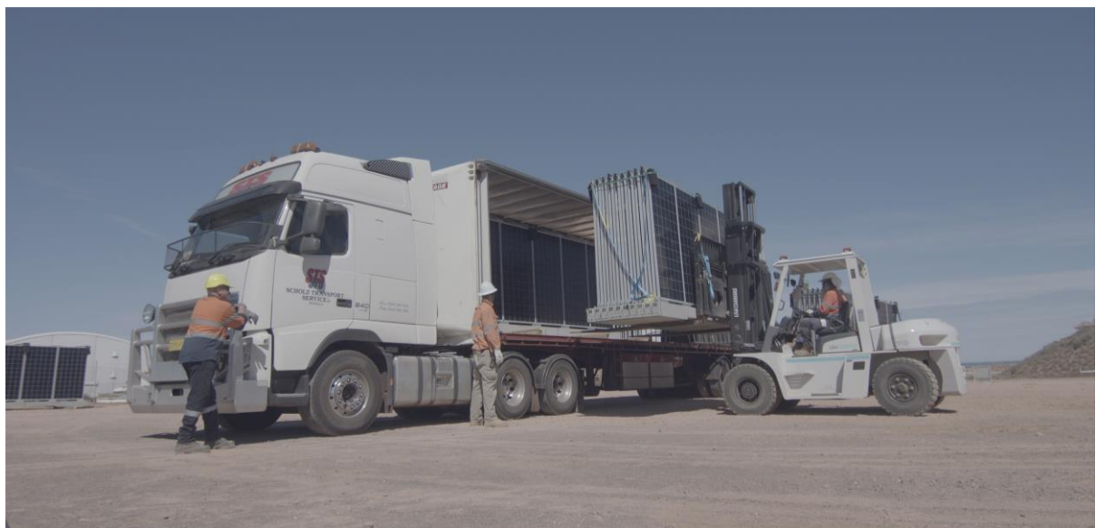
Figure 8. Innovative prefabricated mounting array lowers the cost of deployment in remote regions. Images courtesy of 5B Pty Ltd.
