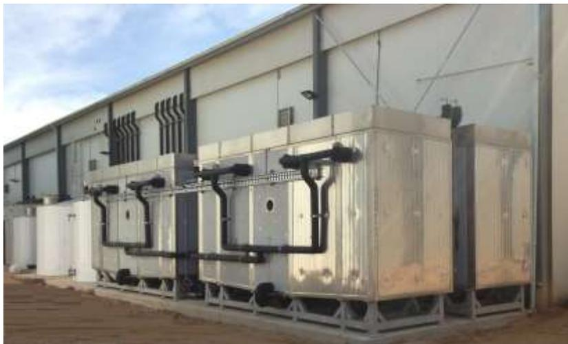
**Figure 2. Thermal storage facility consisting of 4 tanks filled with PCM.**
