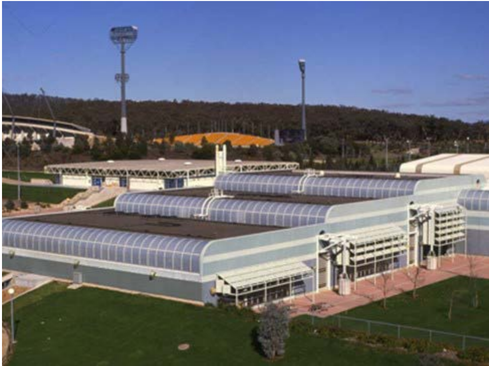
Figure 1 AIS 1500 m 2 unglazed solar heating system (source: Lovegrove 2016)
