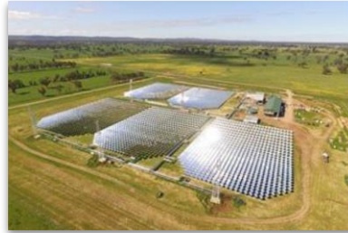
Vast Solar CST plant
