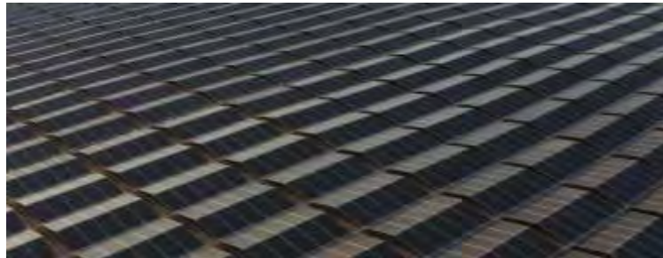
Figure 1. Image of a deployed 5B array in South Australia
