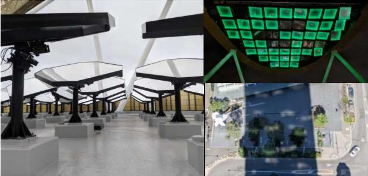
**Figure 1. Rhodes Central heliostat features an array of sun trackers on the building roof, and an array of secondary reflectors on a crown structure above. The heliostat directs light into a nearby park during the day, and has an integrated night-glow feature[1].**
