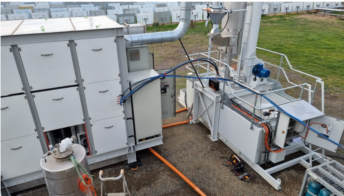
Figure 2. Both the sodium test loop module and wet venturi fume scrubber module connected together at Vast's Jemalong site.
