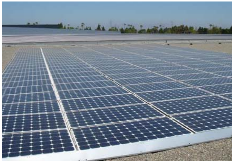
Example of lightweight, insulating, self interlocking PV roof tiles which require no roof penetration (Photo: SunPower - Powerguard®)
