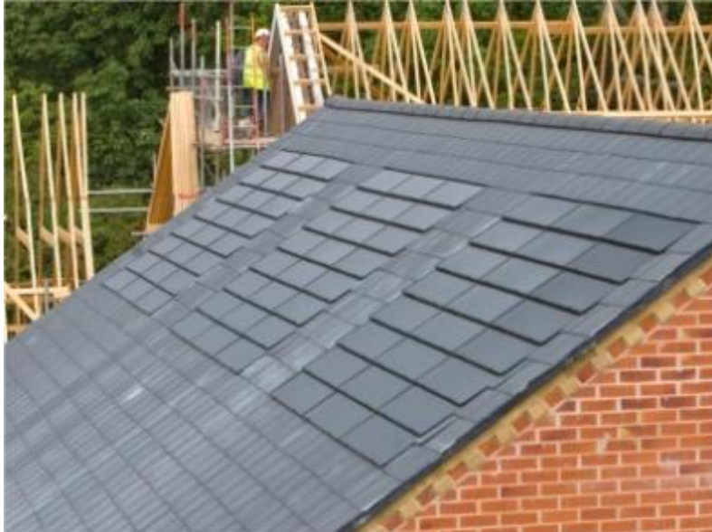
Example of PV roof tiles which blend into a slate roof and may be acceptable in a heritage area. (Photo: Solar Century)
