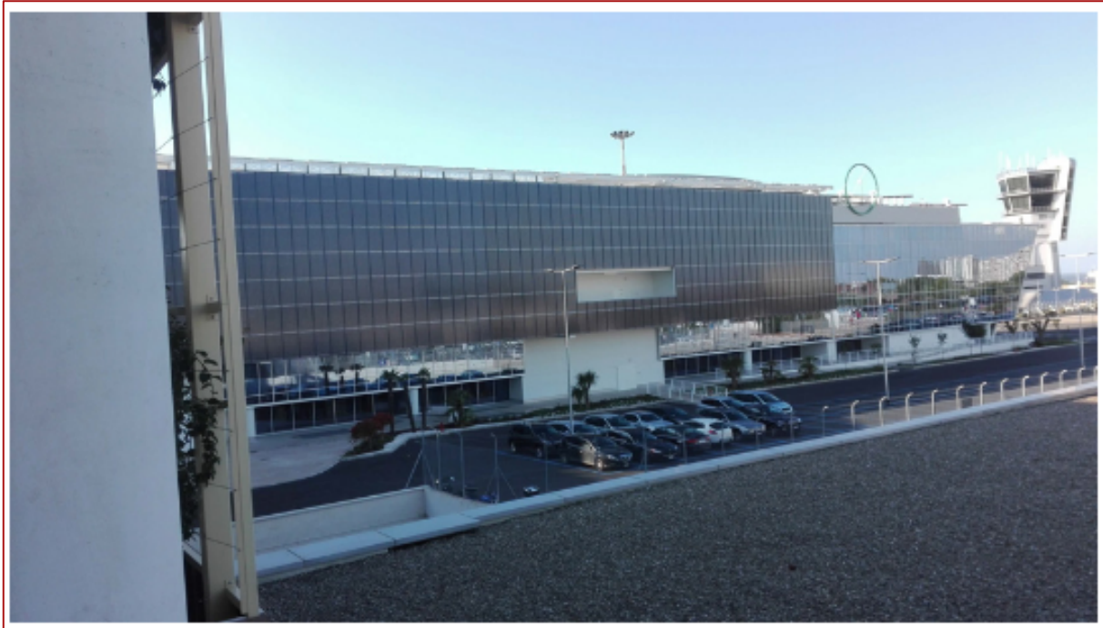
Figure 3: PV façade of the airport terminal of Bari Palese (Mazziotti et al., 2016)
